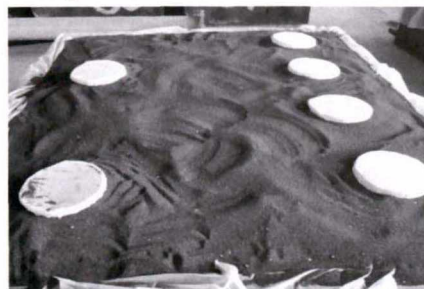
图 30 覆盖薄膜后加保护砂层 Fig.30 Add sand to protect covered plastic film
