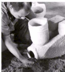
图 24 水玻璃砂填塞缆索孔 Fig.24 Fill the hole of the clip with water glass sand
