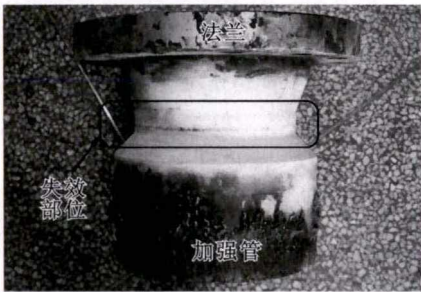
图2 现场截取失效件 Fig.2 Failed part intersepted on site
