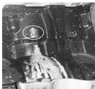
图3 漏水位置 Fig.3 Location of water leaking
